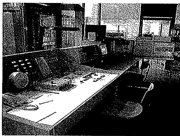
Control station for tests up to 10kA
