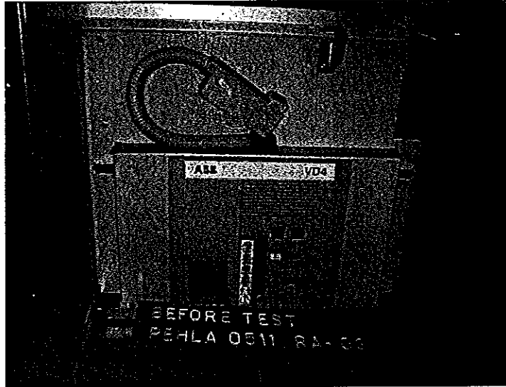
Photo No. 01 Before Test no. PEHLA 0511Ra / 03
