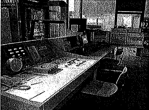
Control station for tests up to 10kA
