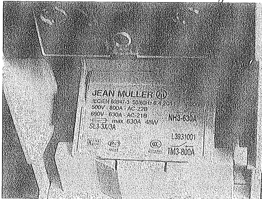
Rating plate of the fuse-switch-disconnector
